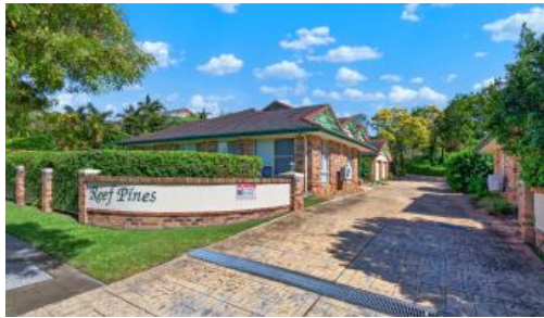
Unit 4, 33 Ward Street, Southport
